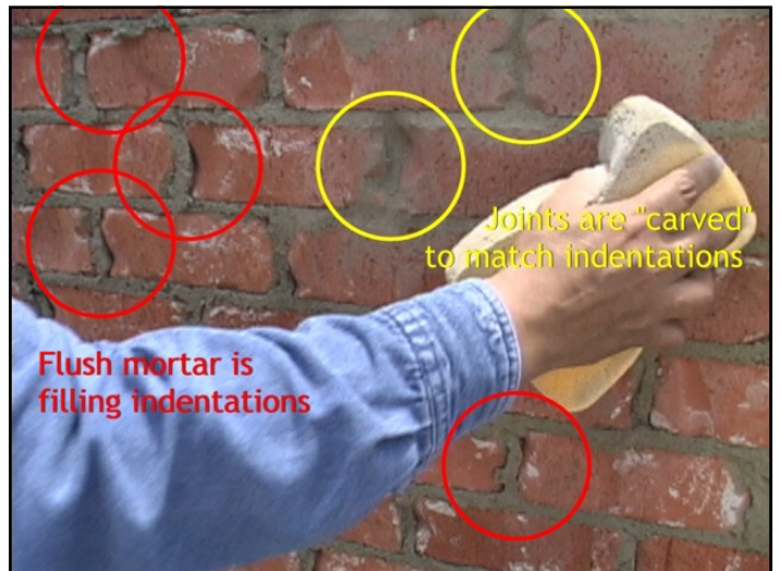
The flush mortar joints are finished with a damp sponge in order to compress the joints and remove the excess mortar in the brick indentations. See highlights below.
