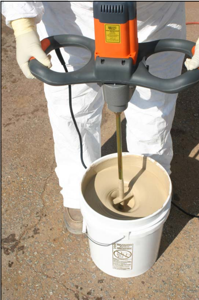
The finishing mix is blended briefly as each pail is opened to ensure no materials have separated during transit or storage.
