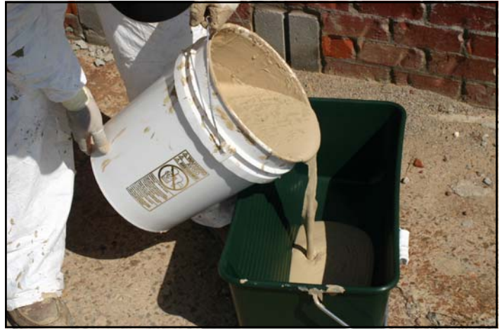
If a roller is used to load material on the wall, then a roller cover with a heavy knap of 3/4" or 1" should be used along with a high-capacity roller pan.
