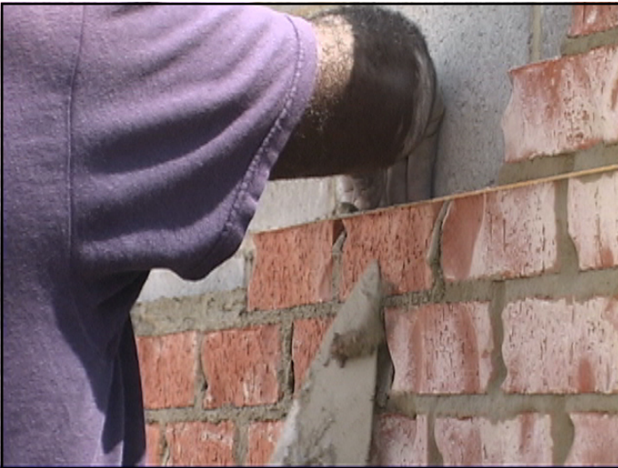
The PastelBrik® brick are laid like any other face brick veneer. The excess mortar is cut from the wall with the trowel.
