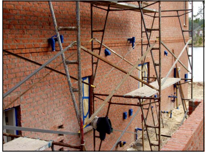
This wall has been well-masked with painter's tape and paper. All piping, electrical wiring and panels, vents, windows and doors should be completely covered.
